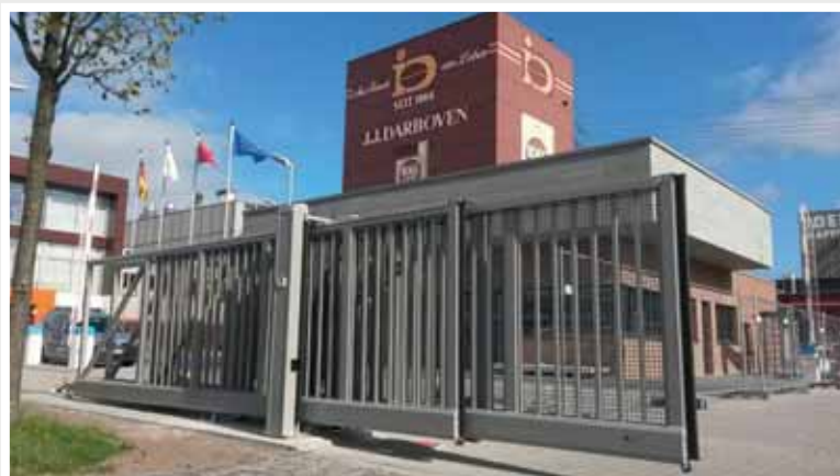
9 m Teleskopschiebetor, Profil 30/30, RAL 7030 Matt, Inline 250-T
